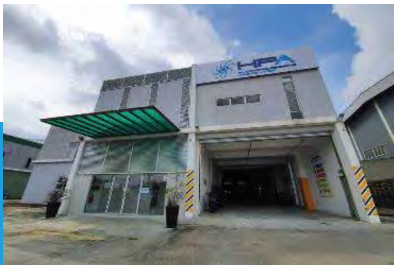
HPA Malaysia Office
